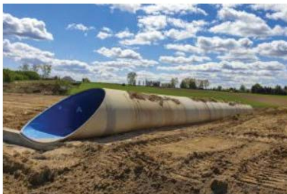
Fig. 9. GRP road culvert with a non-circular profile, dimensions 3000/2250 on the S6 road Szemud – Gdynia, Wielki Kack, Poland [10].
