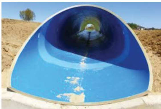
Fig. 9. GRP road culvert with a non-circular profile, dimensions 3000/2250 on the S6 road Szemud – Gdynia, Wielki Kack, Poland [10].
