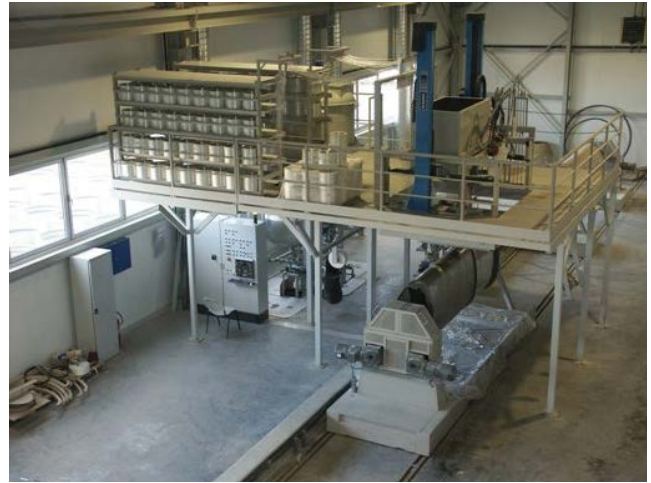
Fig. 5. A typical production system for pipes forming on a mould [10].
