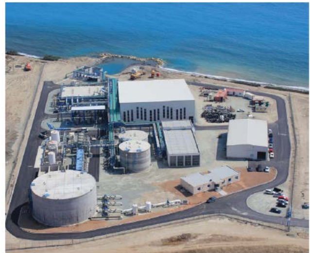
Fig. 2. Air view of Limassol desalination plant. Courtesy of MN Limassol Water Co.
