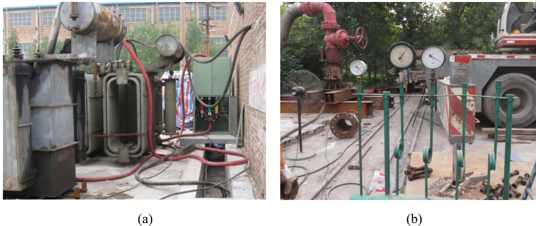
Fig. 12. Submersible pump (a) test process and (b) data recording.
