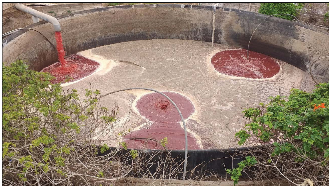
Fig. 1. Storage of meat wastewater in the equalizing tank after pre-treatment.
